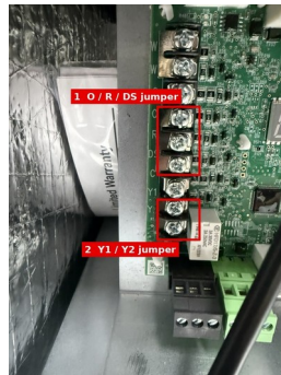
Low-voltage terminal strip. Box 1: O / R / DS terminals. Box 2: Y1 / Y2 terminals.
